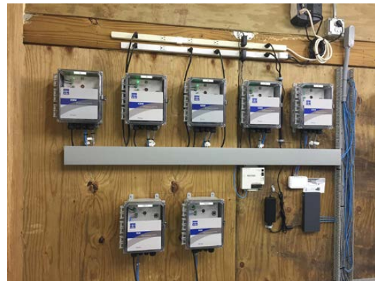
One of the Clusters of YSI IOEM and REM Instruments Providing Continuous and Automated Control.
